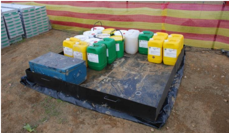
Photo 17: A drip tray is present beneath the stored chemicals.
