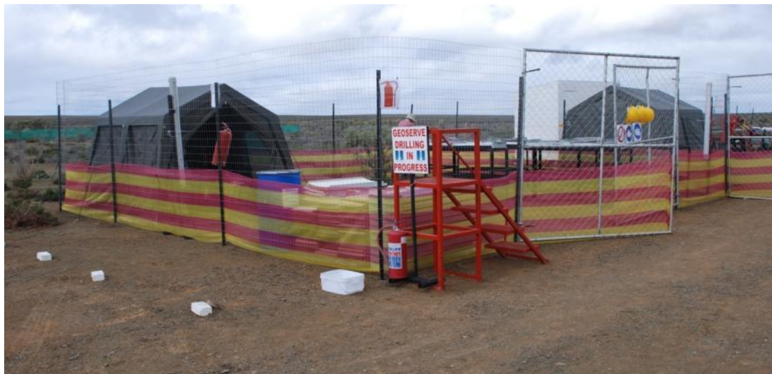
Photo 4: The site has been appropriately demarcated with a security fence and safety netting. The core storage and logging area in the foreground is separated from the drilling area.
