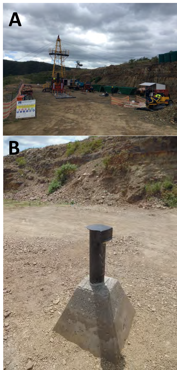
Fig. 3A. Photograph of the drill site in the road quarry near Willowvale. B. Sealed borehole after demobilization at the site.
