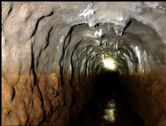
ca. 400 m. Small, soda-straw-type stalactite from spray-concrete roof
