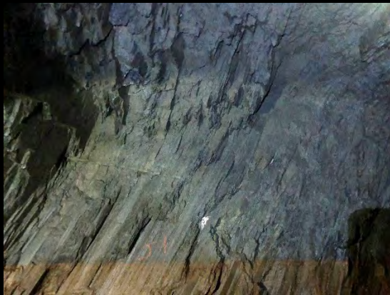
dry walls and ceiling from ca. 2600 m
