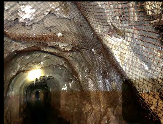
1020 (foreground; wire mesh only) – 1040 (background; U-frames and spray-concrete) m
