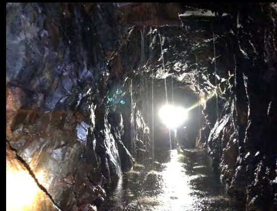
2100 m; dripping water; shallow
