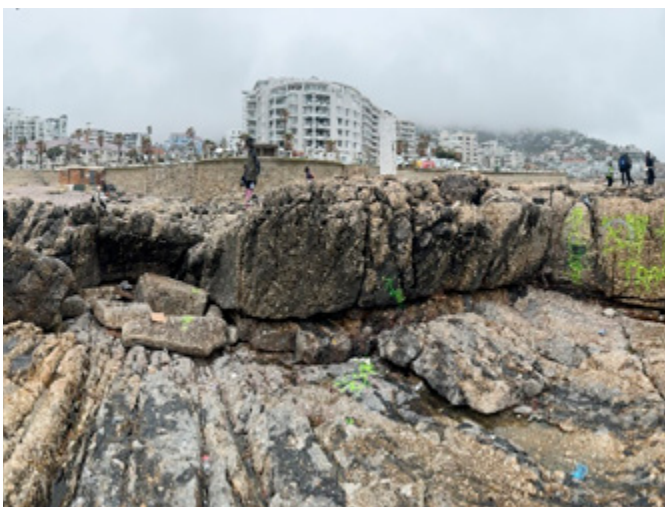
Figure 1: Vandalism at the Sea Point Contact location.
